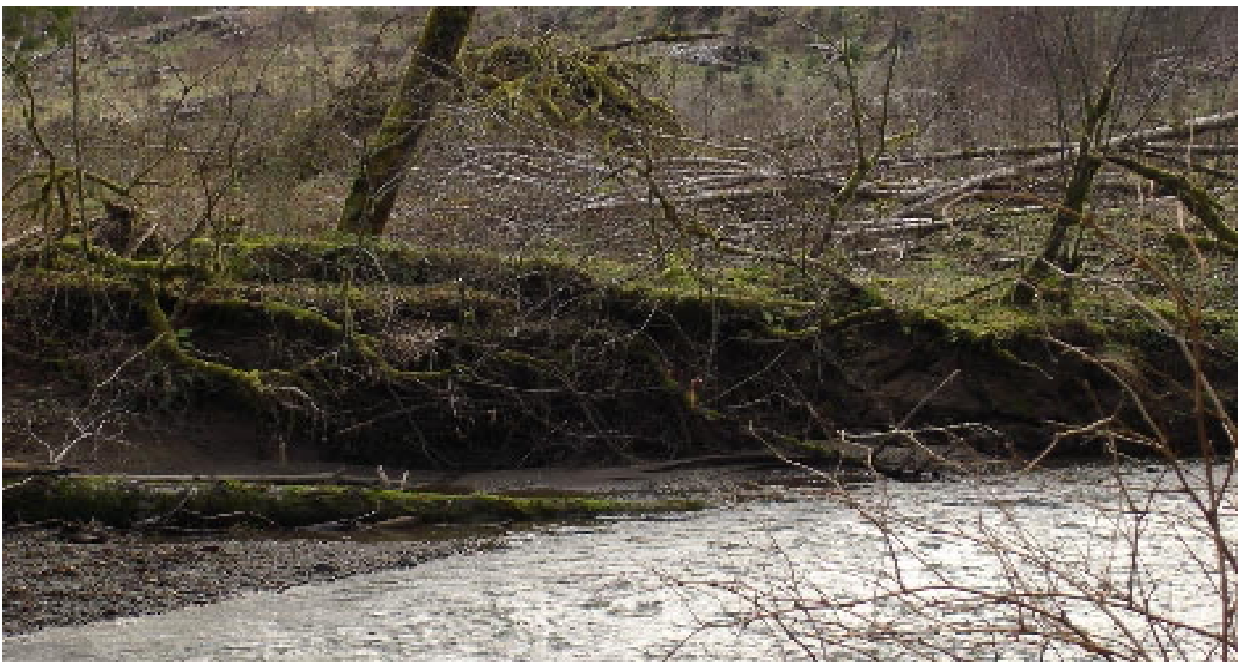
Bank of the Pysht River shows erosion caused by forest practices and skimpy riparian protections.
