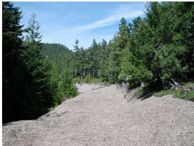
Forest Service Road 2875 above Slab Camp after decommissioning project, successfully re-wilding the Gray Wolf River valley.
