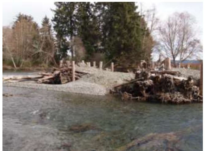
Tons of gravel were used to form this island.
