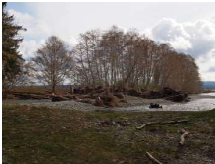
This Engineered Log Jam is located at the Dosewallips State Park, at the river's entrance to Hood Canal. It is readily visible from the campground and picnic area of the beach side of the park.
