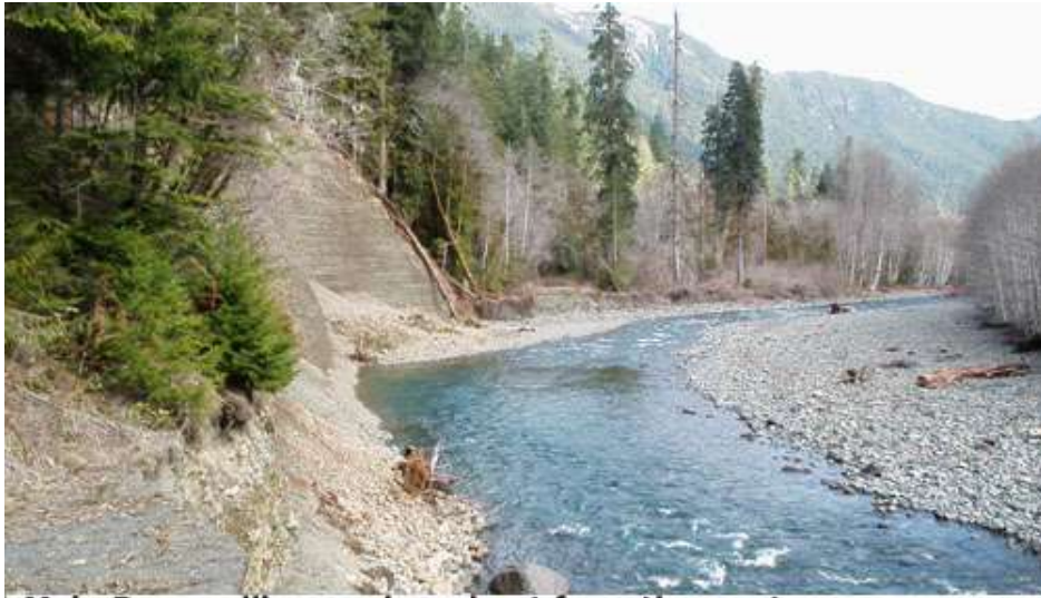
Main Dosewallips road washout from the west. The Forest Service's "instream" reconstruction alternative would build a road directly through the river here.
