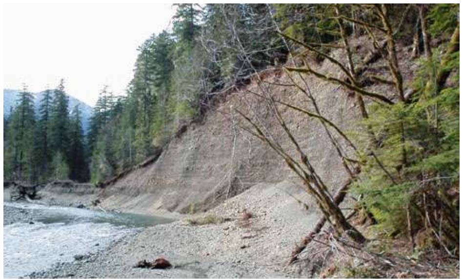
Main Dosewallips road washout from the east. The river now flows where the road once was.
