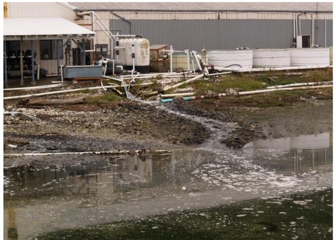
*This picture of the Coast Seafoods facility shows many of the pipes, ditches and channels it uses to discharge effluent to Quilcene Bay.*
