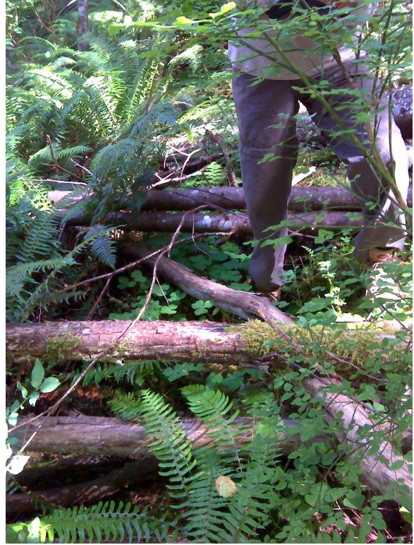
A33-3B N47 35.398 W124 01.929 Notes: Large fissures in road Direction: 360°
