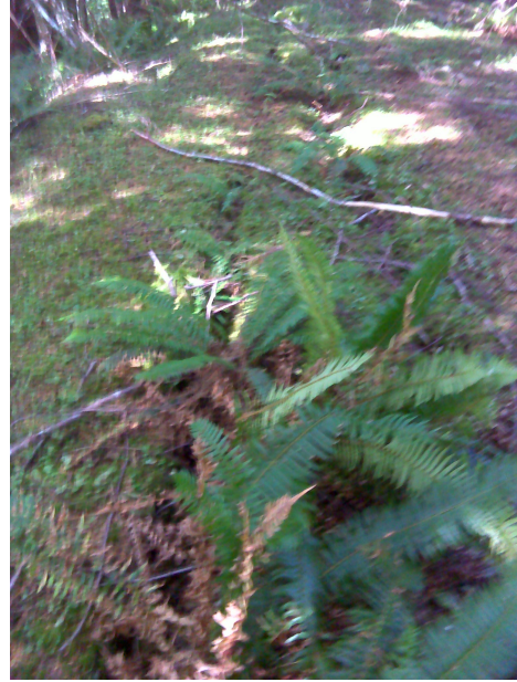
A33-2B N47 35.251 W124 01.975 Notes: Large tension cracks, severe slope failing and holes Direction: 230°
