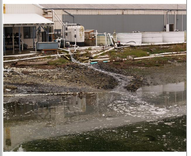
The point sources at the facility include the many pipes discharging onto the beach and into Quilcene Bay; the man-made and eroded channels discharging onto the beach and into Quilcene Bay; and the facility's seawater intake pipe, which discharges when the facility back-flushes that pipe. Effluent added to Quilcene Bay from pipes, ditches, and channels at the facility is not "non-point source pollution."
